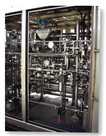
The plants can be supplied on skids or turnkey assembled inside ISO transport containers. All components are selected according to the environmental conditions and the installation site classification.
